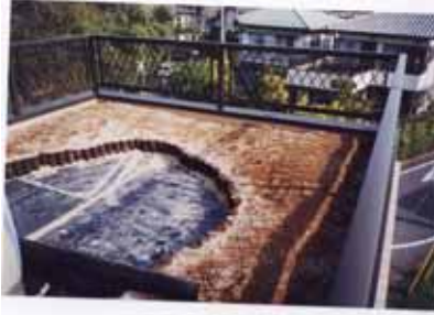
Putting soil on Porous Alpha
