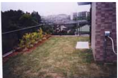
Planting lawn Completion
