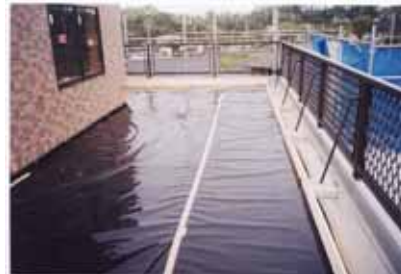
Setting water-proof sheet and draine
